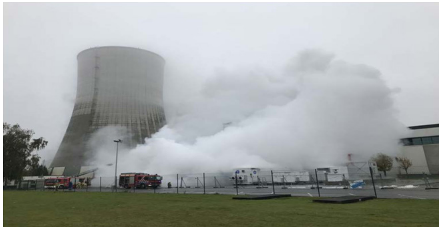
Figure 22. 2017 fire at an Engie Ineo BESS facility in Belgium (IMIA Report Photo)
