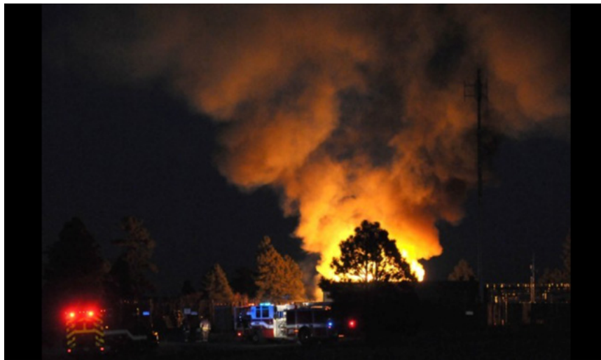
Figure 19 The 2012 BESS electrical fire at the Arizona Public Service facility near McMillan Mesa (Josh Biggs/ Arizona Daily Sun)
